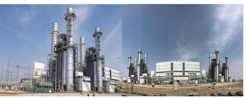
The combined-cycle power plant is a next-generation facility. Four 9 FA gas turbines, four waste heat boilers designed to generate steam, two steam turbines and other equipment will be installed at the new power plant.
