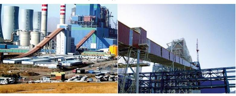
Afşin-Elbistan B coal fired power plant has fully automated conveyor systems feeding power plant with coal and transferring waste -ash out.
