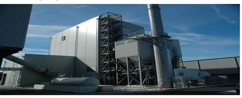
The chicken litter-fired and environment friendly power plant will produce 35 MWe in Turkey. Boiler capacity: 99.5MWth, 92 bara, 472°C, Electrical power ≤35MWe
